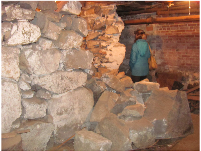
Right: Part of an interior foundation wall collapsed.
