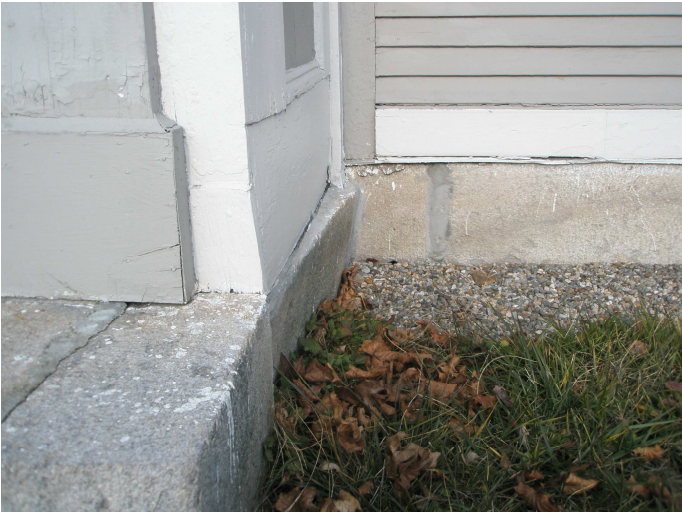
Left: The foundation underpinning is leaning outward.
