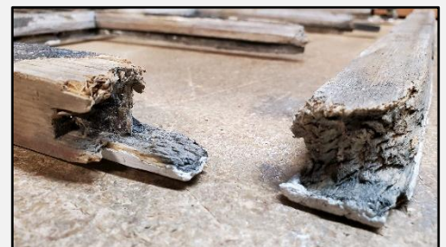
Close-up of wood damage
